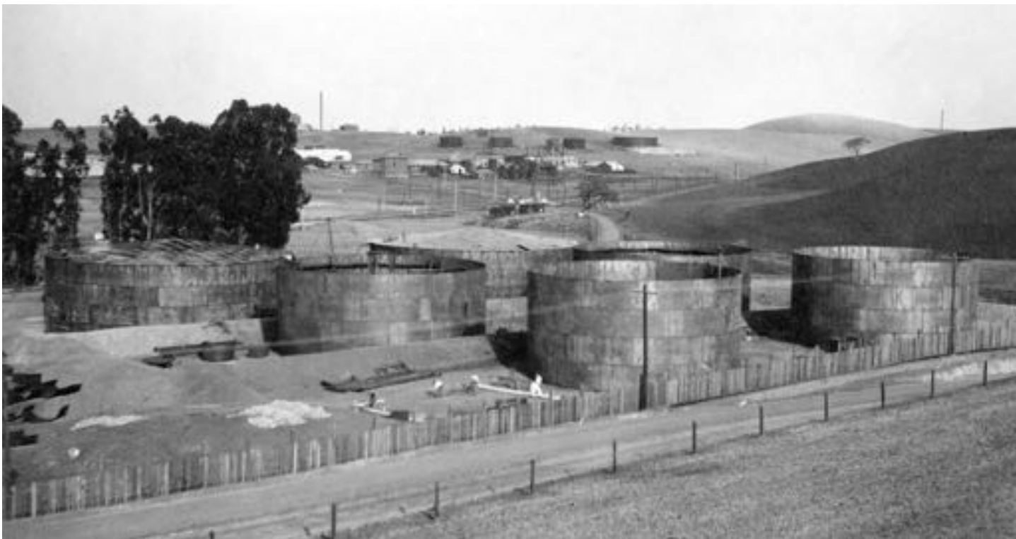
Six tank under construction. All sides completed, tank #1 & #2 to rear have roofs installed. The American Occidental refinery visible behind the row of trees. View looking north east. December 15th, 1912.
