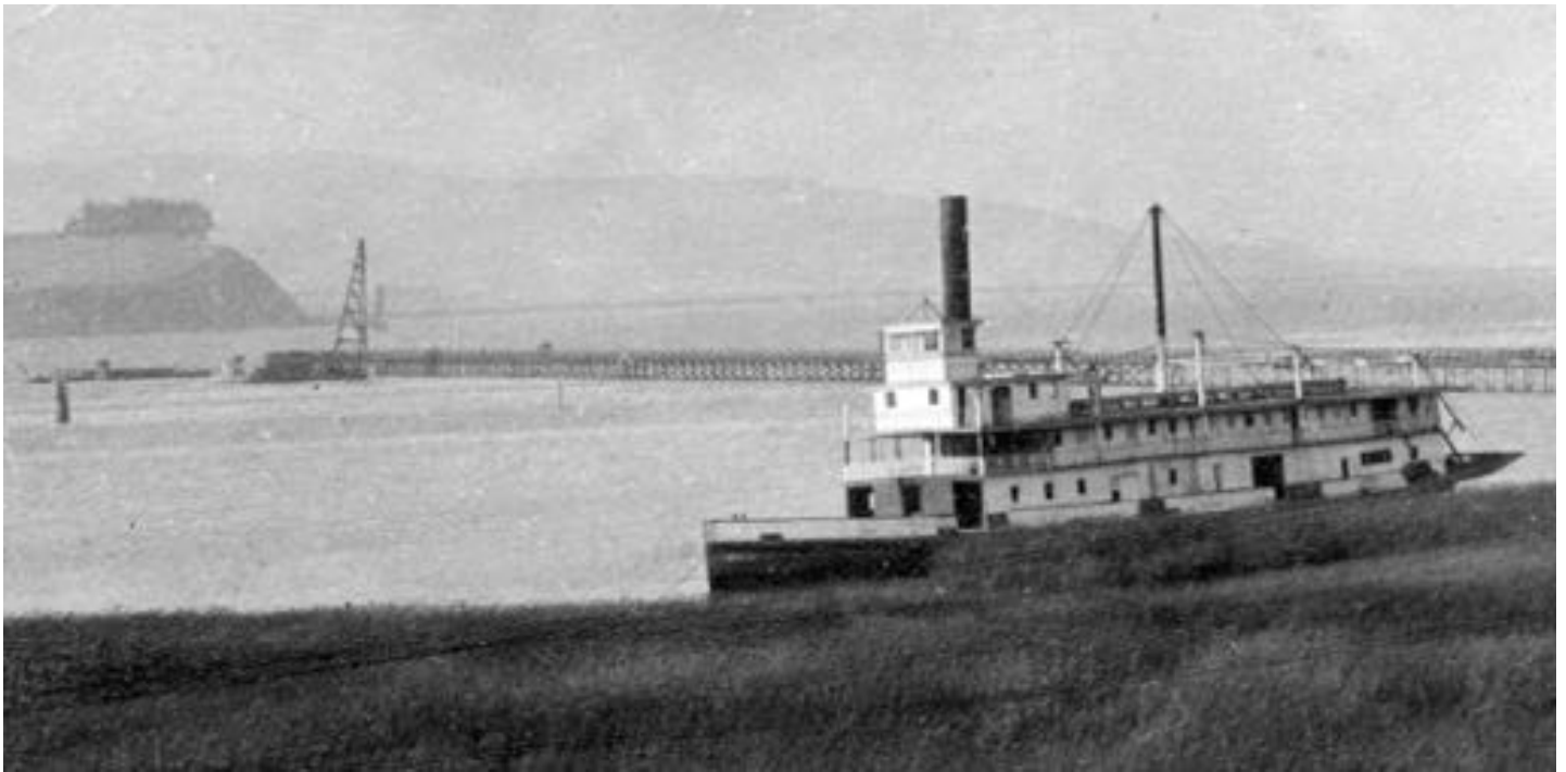
View of the new wharf looking north from the SW edge of the new Shell Terminal property. Old SP Ferry Steamer "ONWARD" in mud flat in front of new wharf . Crane finishing Wharf and setting piles for the new Wharf Boiler House. September 27th, 1912
