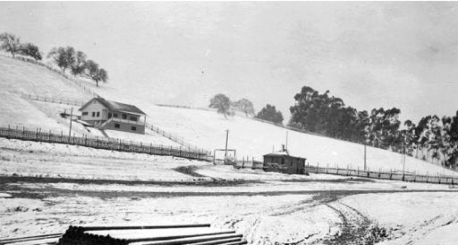
Office, gate and Bungalow covered in snow. View looking South West. January 8th, 1913.
