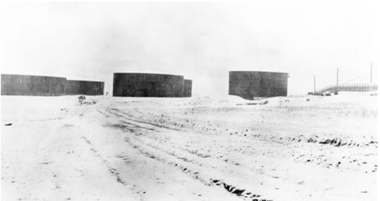
The six tanks covered in Snow. View looking East from Office. January 8th, 1913
