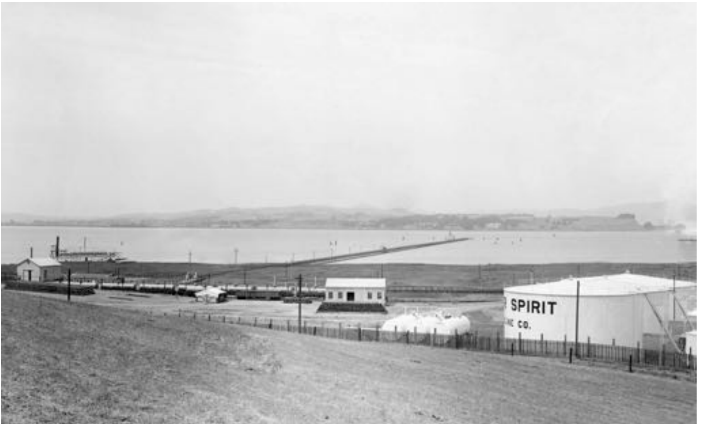
Panoramic view of the new Tank Farm Area from hill across road, looking North-West. Far left boiler house, Dormitory with train of tank cars on siding by loading rack. Filling Shack center in front of tank cars. Tank #5 by fence with SHELL MOTOR SPIRITS on tank. (Photo not in scrapbook.) June 16th, 1913
