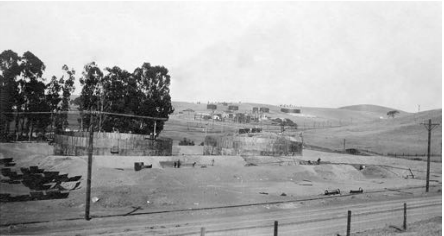
View looking north, Tanks #1 thru #4 under construction. American Oriental Company refinery in background. October 30th, 1912.
