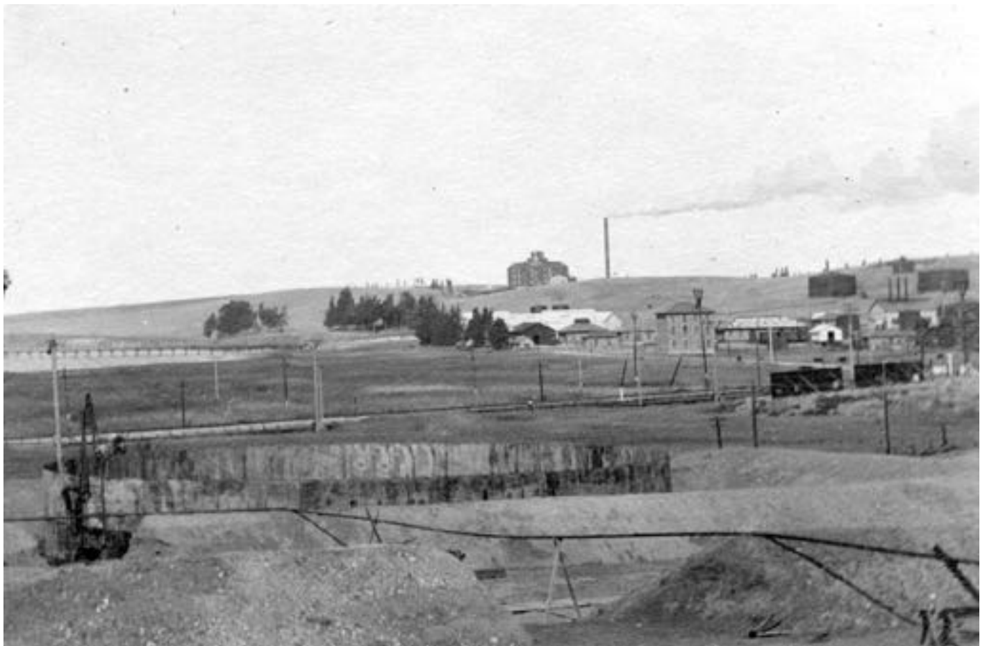
The tanks in various stages of construction. Tank #1 with on the ground and starting row of plates, Tanks #2, with two tiers of side plates installed. View North with American Oriental Co. Refinery and their wharf. Detail of refinery and tank #2 shown below. Mountain Cooper Smelter in hill behind refinery with main building and tall smoke stack. October 23rd, 1912
