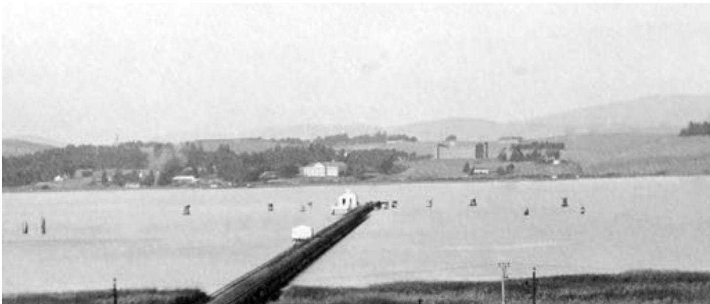
Detail from below. Wharf with pump house and boiler house. View across river showing Benicia Arsenal buildings. December 21st, 1912
