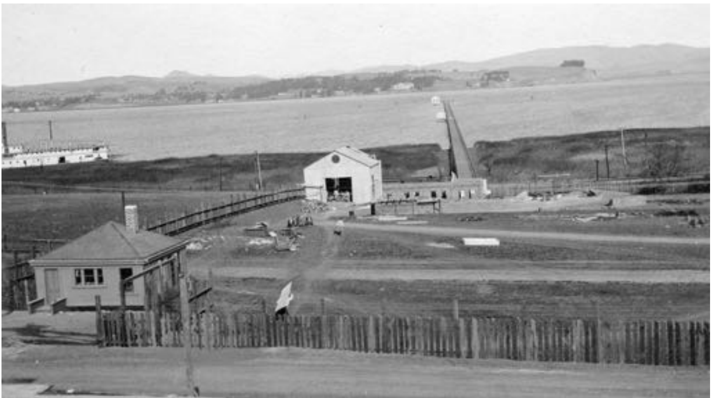
Panorama view office foreground, 30' x 30' Boiler House and Dormitory under construction, Wharf with two buildings. View of Benicia across river looking North. December 5th, 1912.
