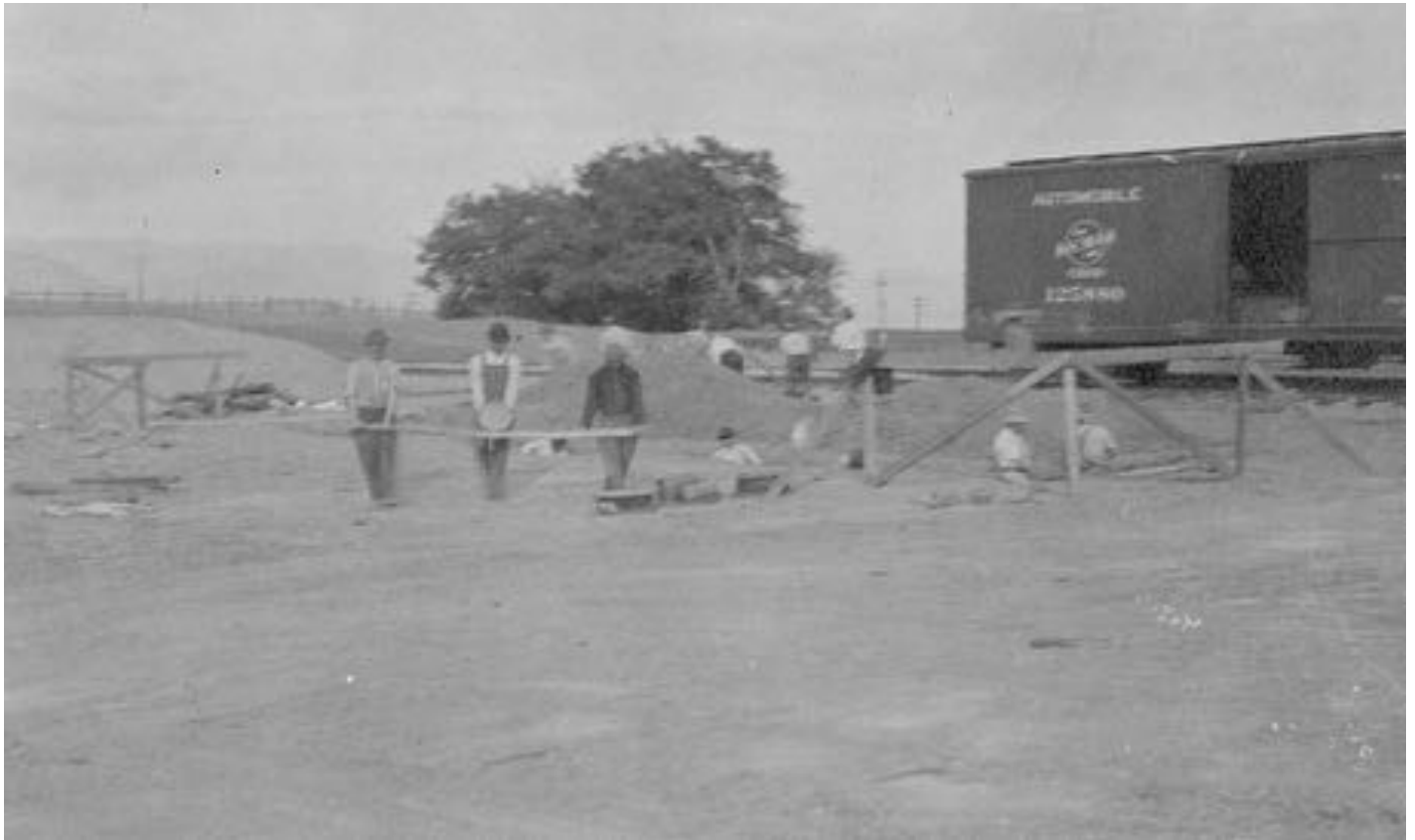
Unloading Material for Filling Shed — View looking North West — September 25th, 1912
