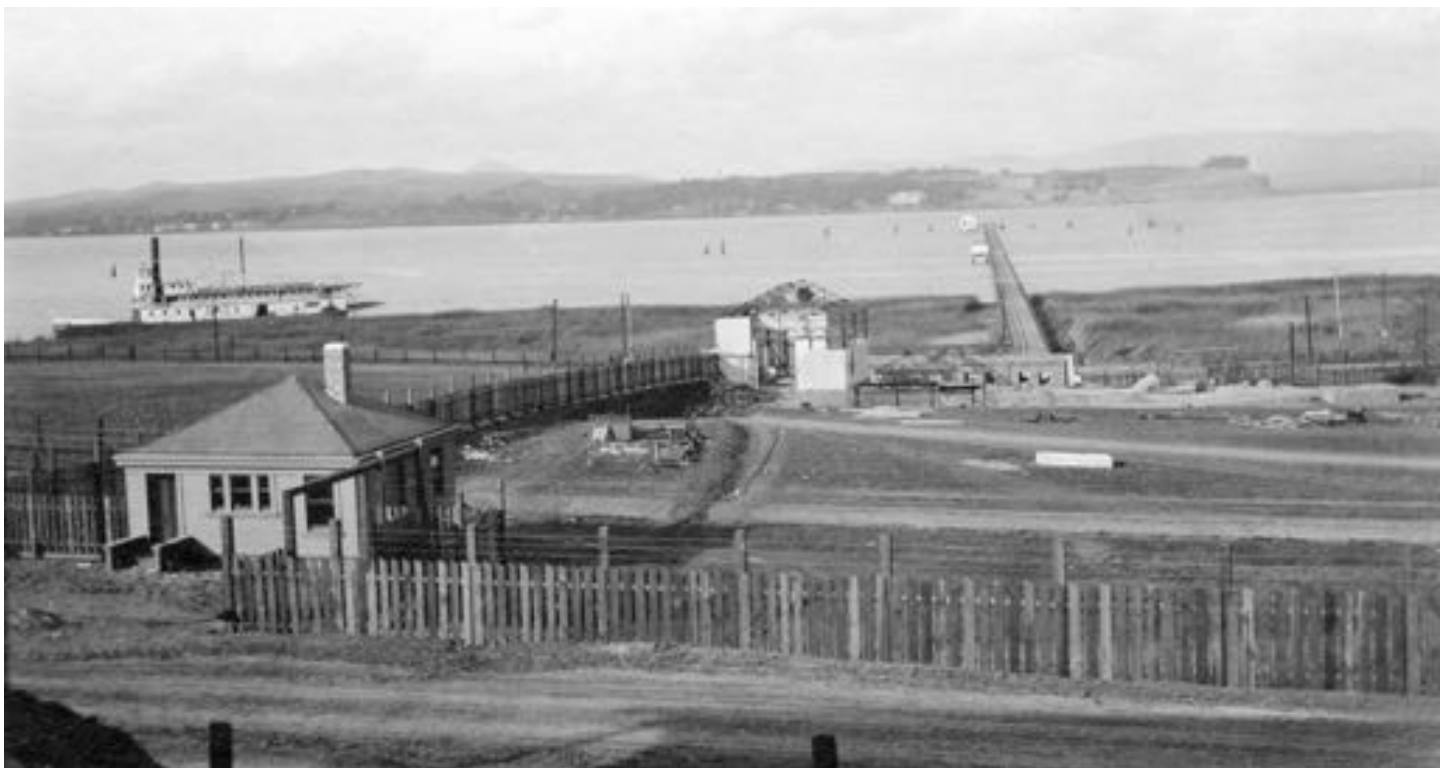
Office in place, Boiler House under construction, and Dormitory. Wharf with Pump House and Boiler House. View looking North. December 1st, 1912
