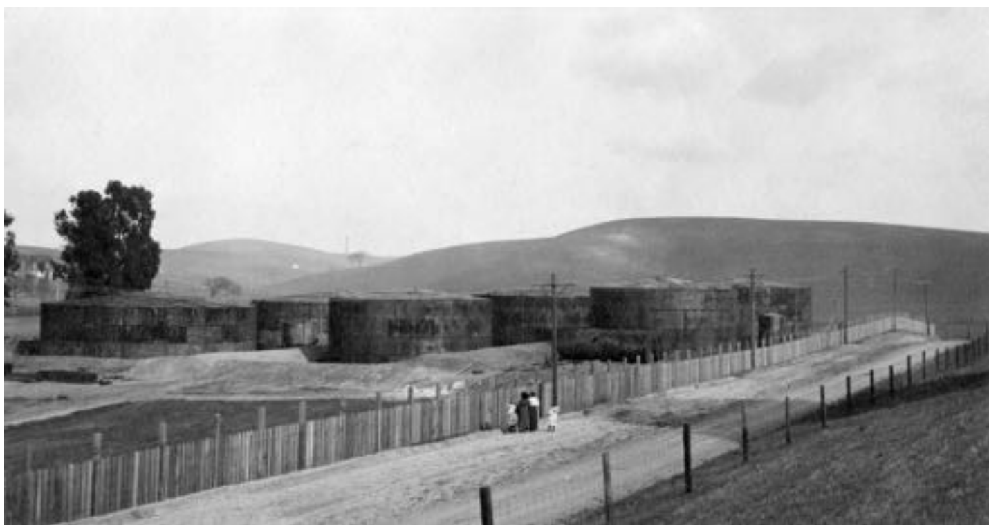
The six tanks with roofs installed. Family looking through fence at progress. Could be talking to worker. Road between the two fences is future Marina Vista. February 9th, 1913.
