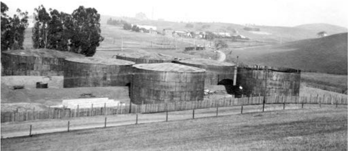
Five Tanks with roofs, Service tanks foundation north west of tank #5. View looking North East. With the American Oriental Company refinery in background and Mountain Cooper smelter in far distance. January 2nd, 1913
