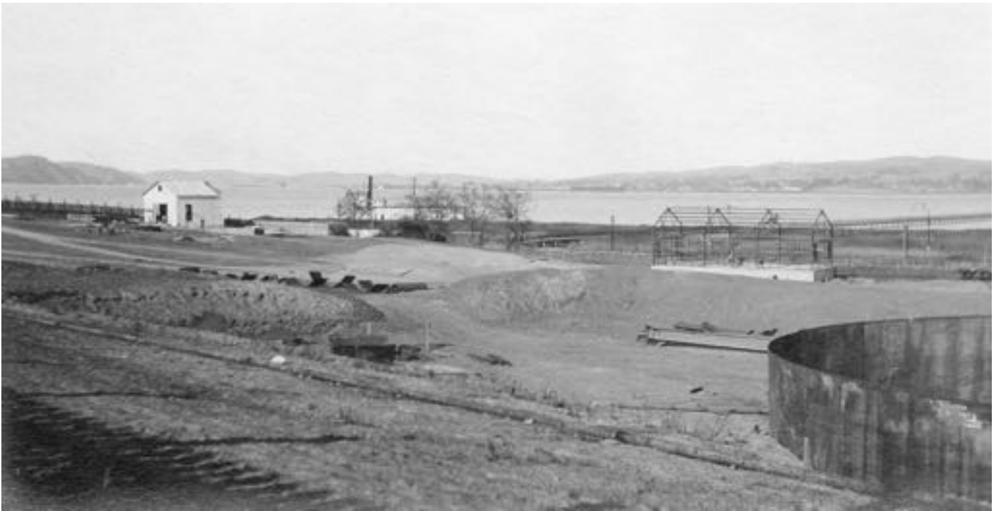
Panorama View looking North West. Boiler House, Start of Filling Shed and 1st pass of side on Tank #5. View of river with end of Wharf looking North West from fence at road. December 5th, 1912
