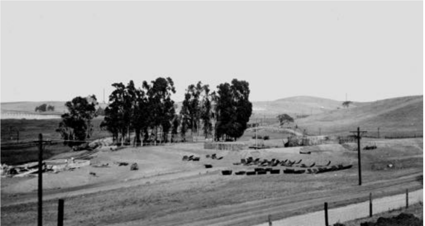
Filling Shed under construction beside tracks on the left. Tank #1 and Tank #2 under construction on the right. The American Occidental refinery and their wharf visible behind the row of trees. View looking north east. October 23rd, 1912.
