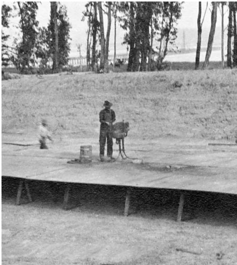
Start of construction of Tank #1 bottom. Tanks were riveted and bottom was raised so rivets could be closed from below. Man standing on center of bottom has a small forge to heat the rivets just before placement. September 27th, 1912.
