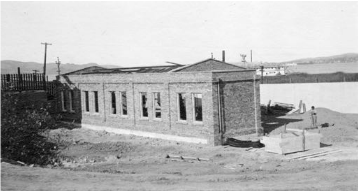
Dormitory under construction. View looking north west. December 5th, 1912.
