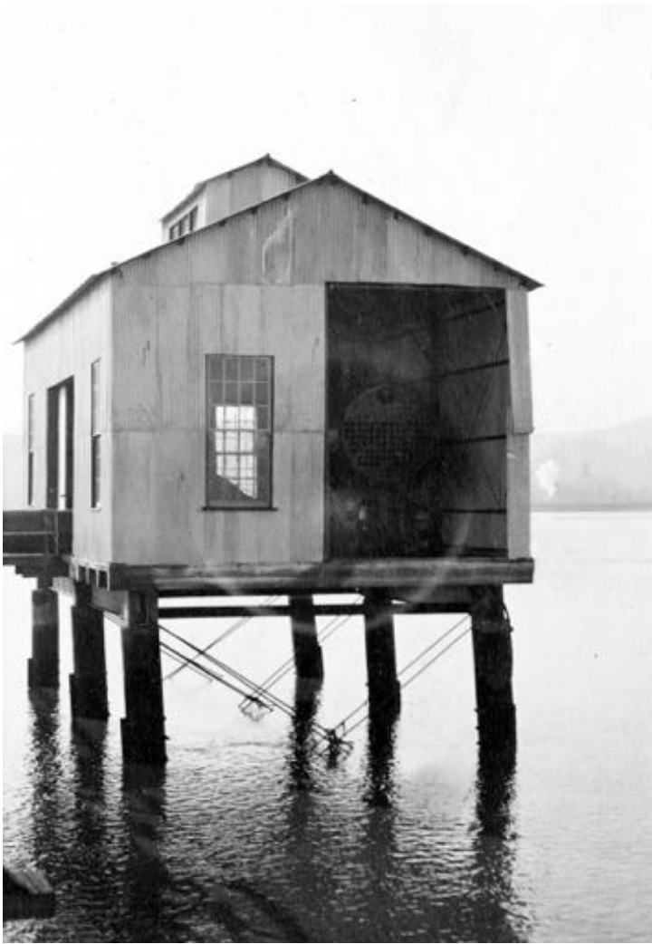
Right: Finished 25 ft x 45 ft Wharf Boiler House with boiler. View looking south west from west side of wharf. January 24th, 1913.
