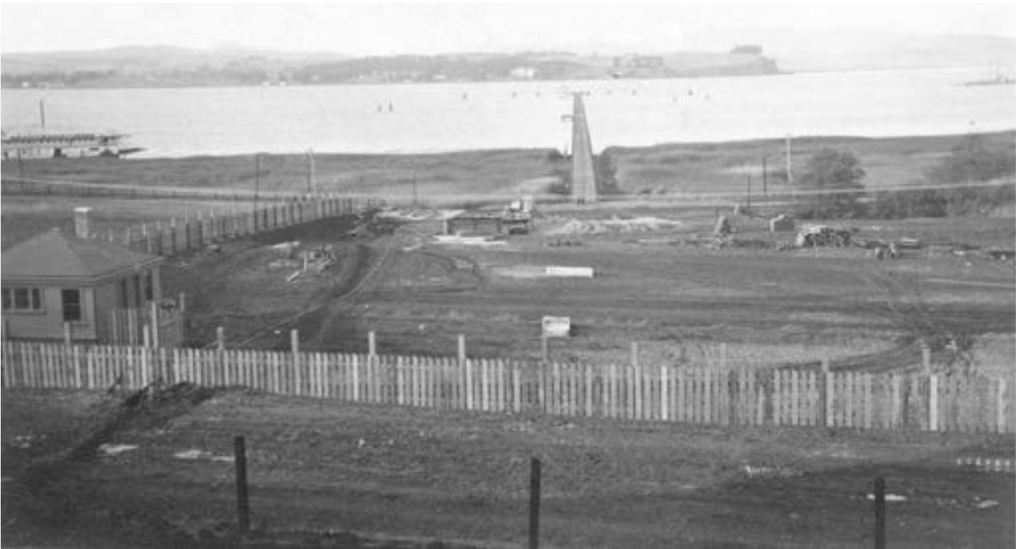
View looking north west. Office building left corner of fenced area north side of the main road. New boiler house foundation under construction. Wharf center, rear of photo. Docked Santa Fe Ferry "Onward" left rear. November 10th, 1912.
