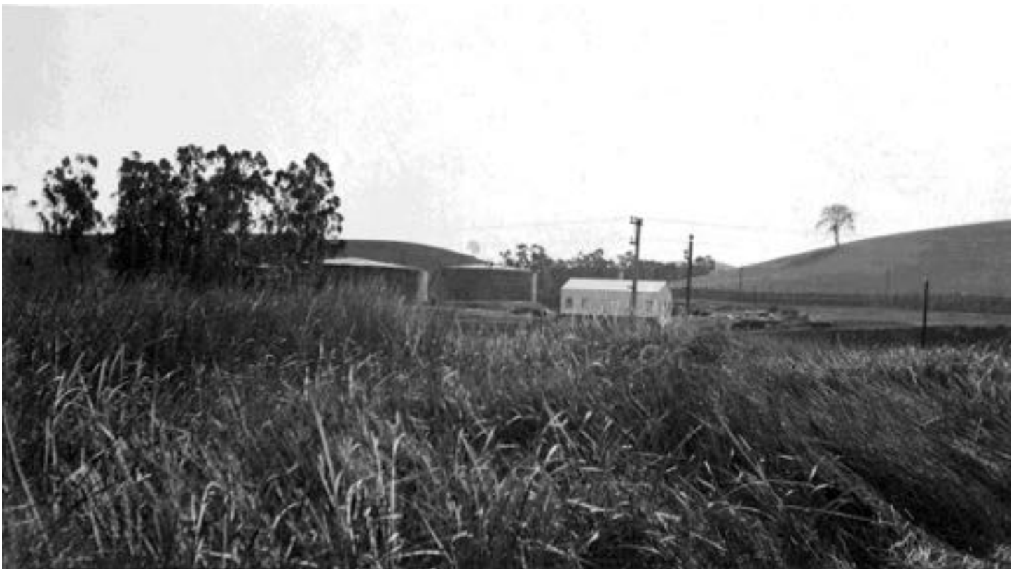
Filling Shed and Tanks view from wharf. View looking East. December 15th, 1912
