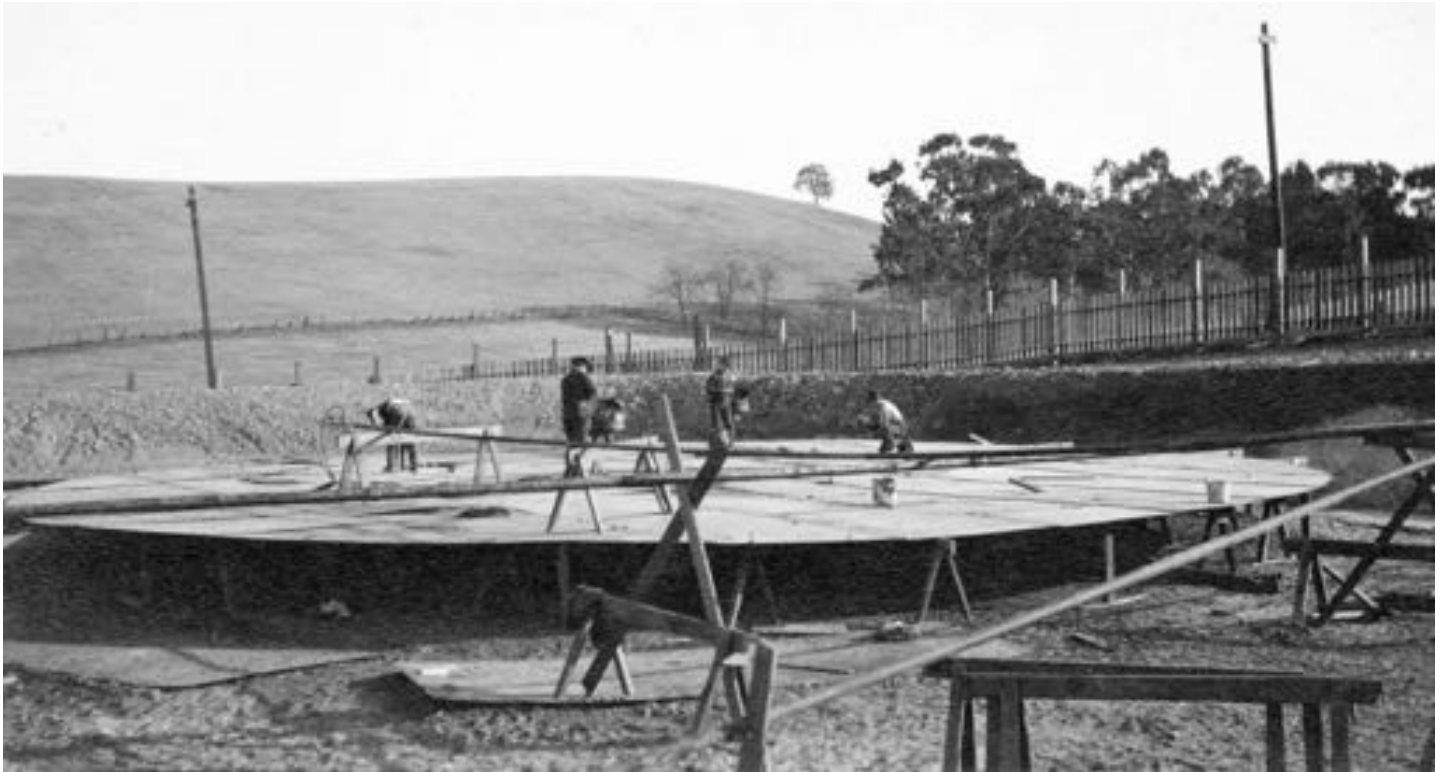
View looking East. Bottom of tank #6 being riveted. Two men with forges and two men inserting rivets in to tank bottom. There are two men under the bottom plate to help in the riveting operation. Road is on the other side of fence. Land in the background is still ranchland and had not yet been purchased for the new refinery. November 11th, 1912.
