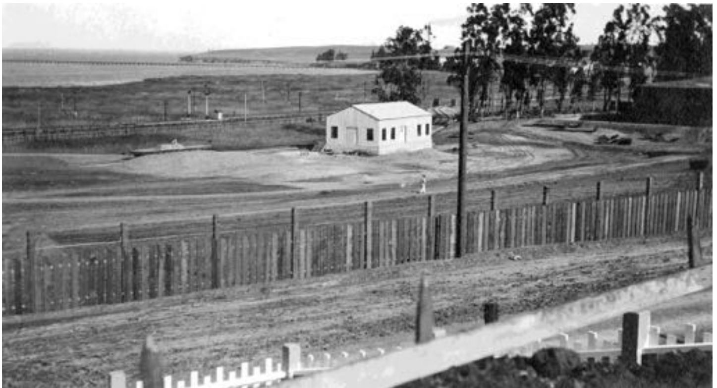
Filling Shed, railroad siding and part of Tank #1 with roof installed. Tanks View looking North East with American Oriental Refinery wharf in distance. December 21st, 1912
