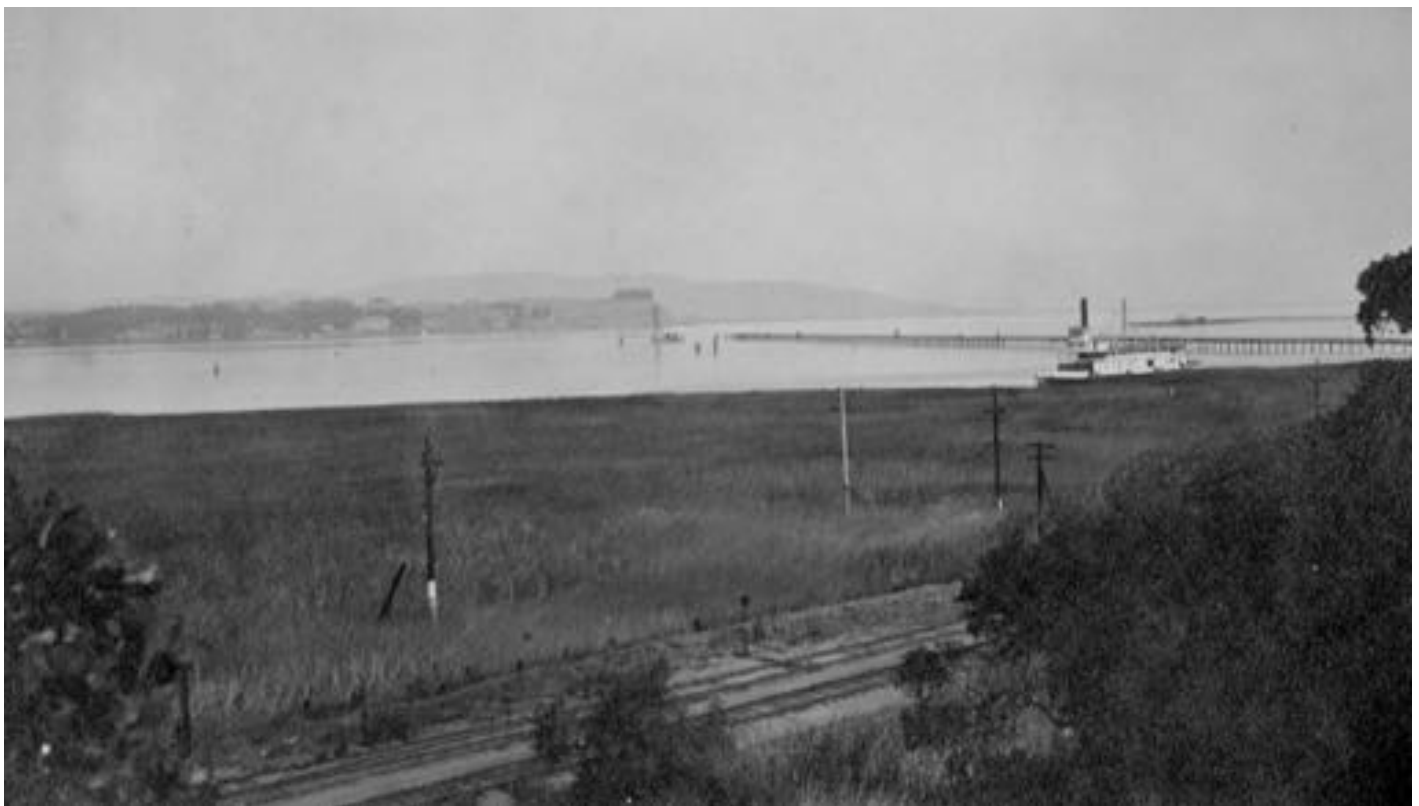
View of the new wharf looking north from the SW edge of the new Shell Terminal property. The main line train tracks in foreground. September 21st, 1912
