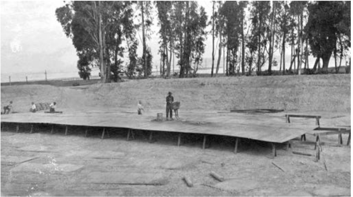
Start of construction of Tank #1 bottom. Tanks were riveted and bottom was raised so rivets could be closed from below. Man standing on center of bottom has a small forge to heat the rivets just before placement. September 27th, 1912.
