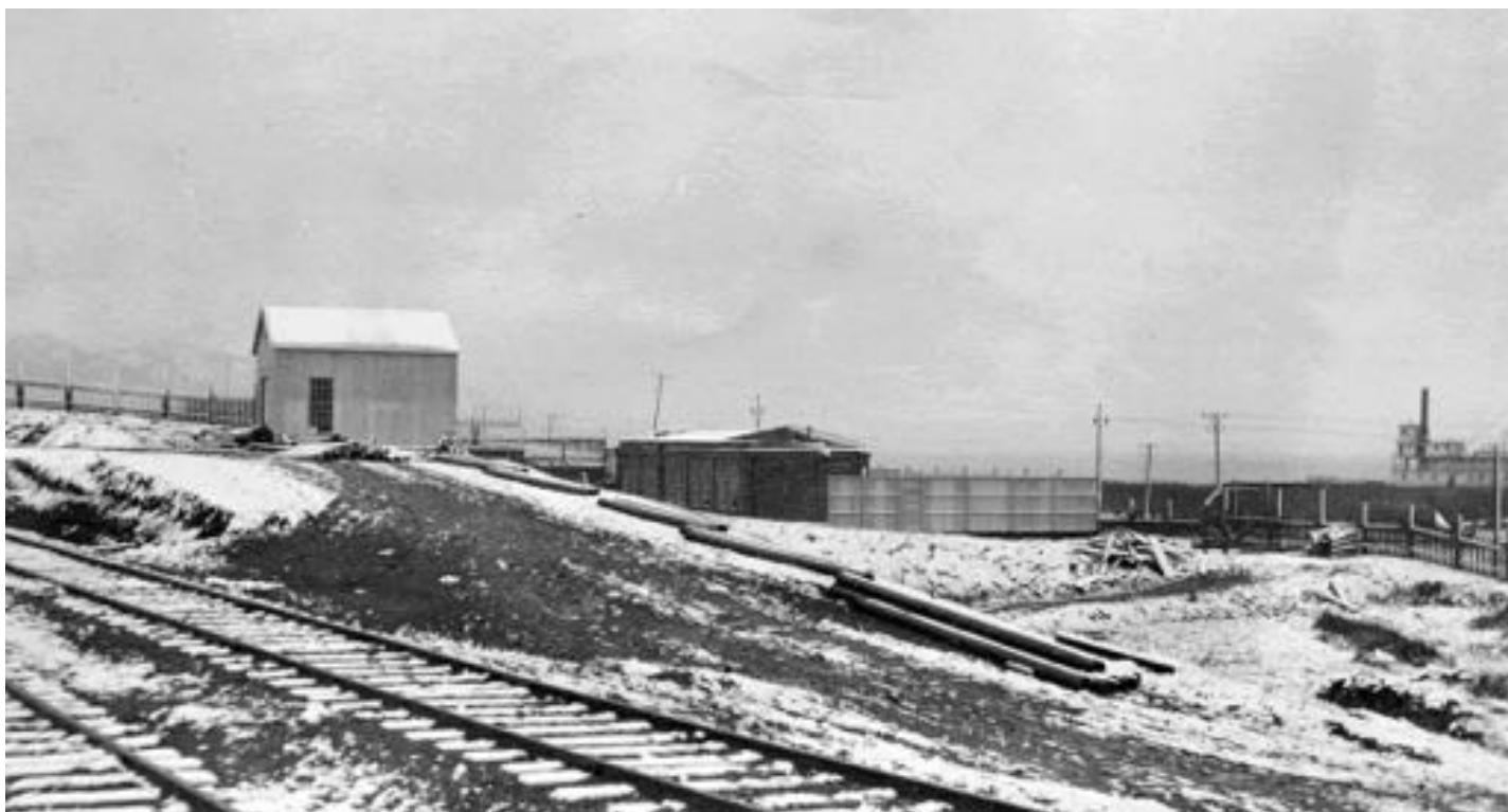
View of Dormitory and Wharf End 30' x 30' Boiler House in Snow. View looking West. January 8th, 1913.
