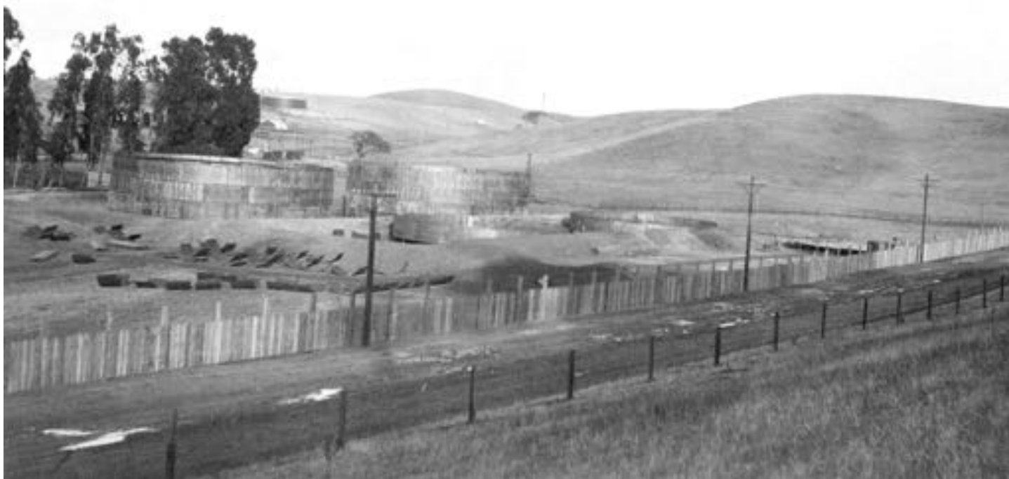
View looking north east six tanks in various stages of construction. Road in foreground will become Marina Vista. American Oriental Petroleum behind trees on left. November 10, 1912.
