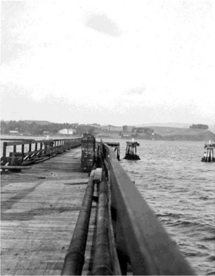
View of Wharf looking North from Boiler House. Benicia Arsenal building across river from wharf. January 17th, 1913
