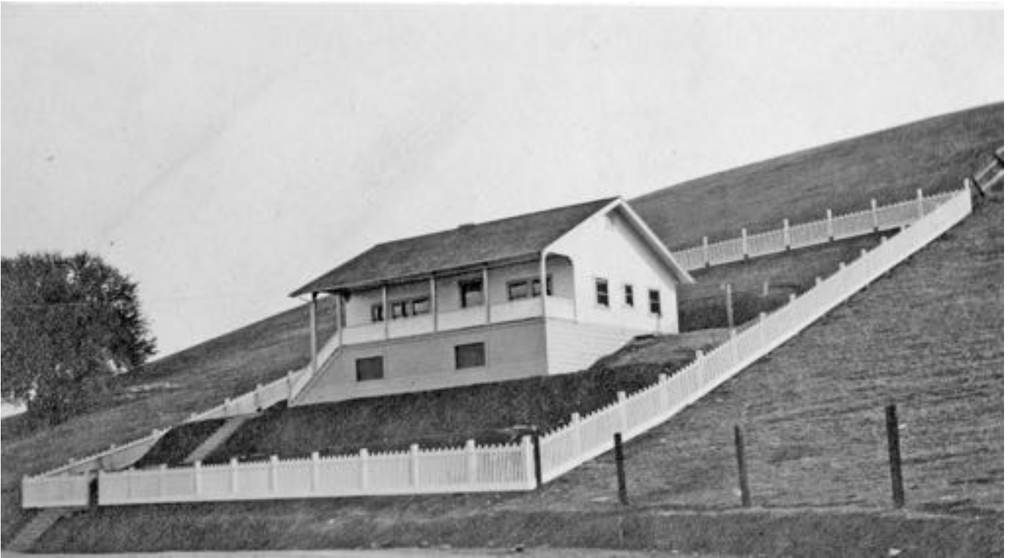
Finished Manager's Bungalow. View looking East. January 2nd, 1913
