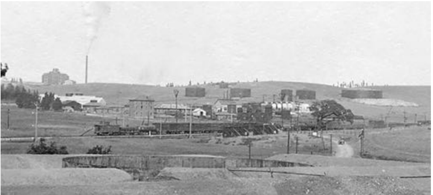
Detail of second tier Tank #2, train on mail line track with view of American Oriental Refinery and the Mountain Copper Smelter in the far distance. View looking North East. November 11th, 1912.
