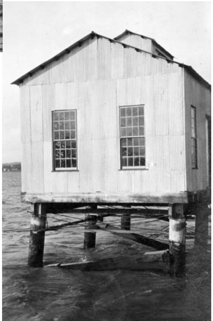
Finished 25' x 45' Wharf Boiler House. View looking North from west side of Wharf. January 17th, 1913
