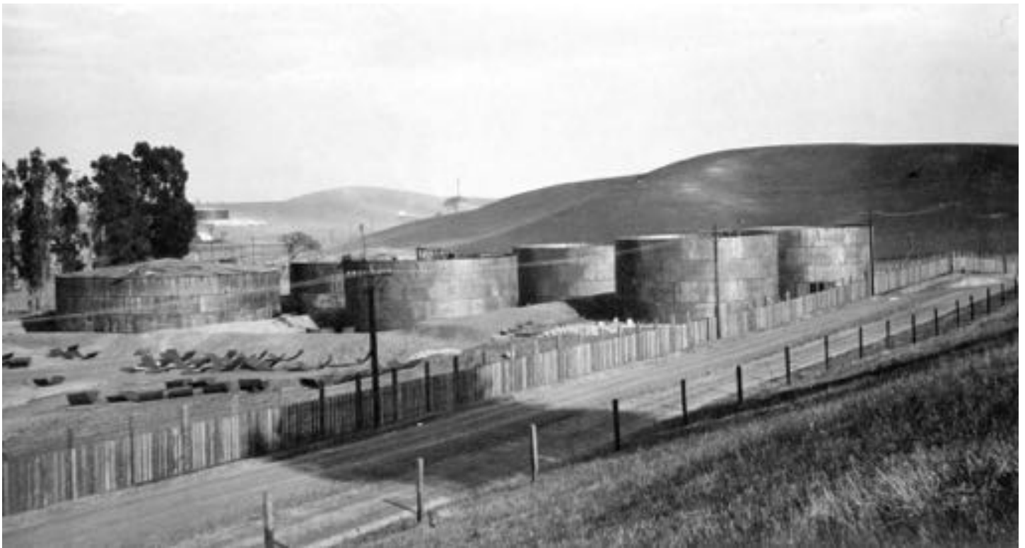
Roofs being installed on tanks. View looking north east. December 15th, 1912
